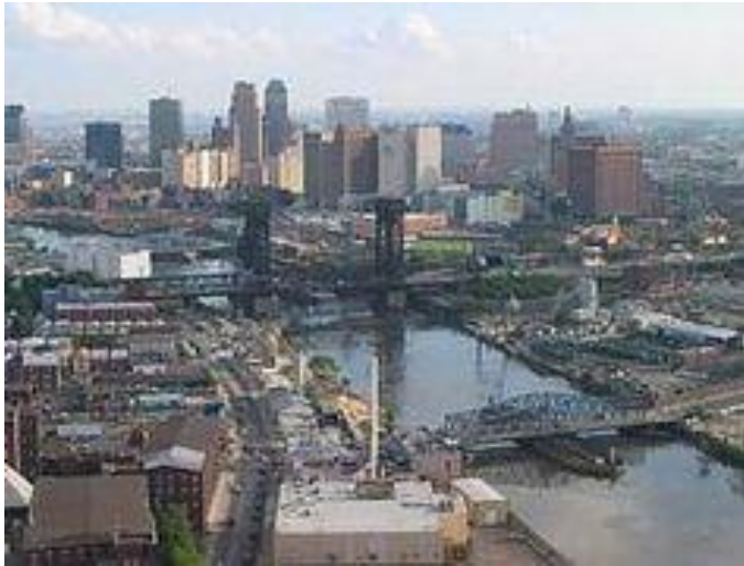
Aerial view Passaic
